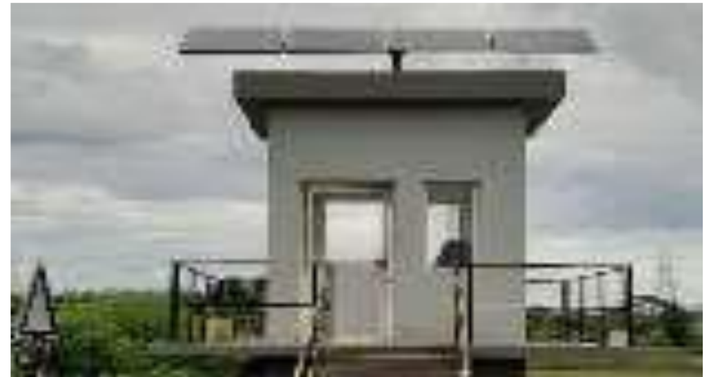
Solar panel at security post
